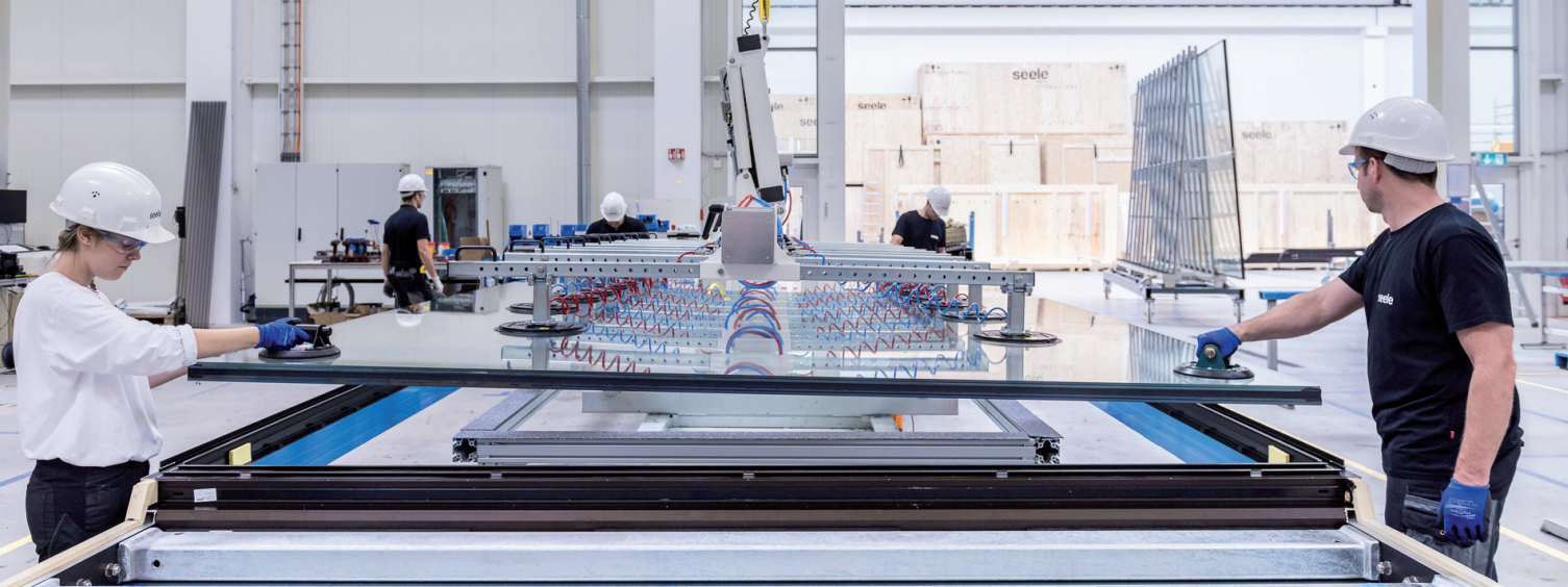
Assembly of up to approx. 7 x 4 m SCF elements for the Principal Place Commercial in London. (Courtesy of René Müller, seele GmbH) Front cover: The Principal Place Commercial in London. (©seele)
